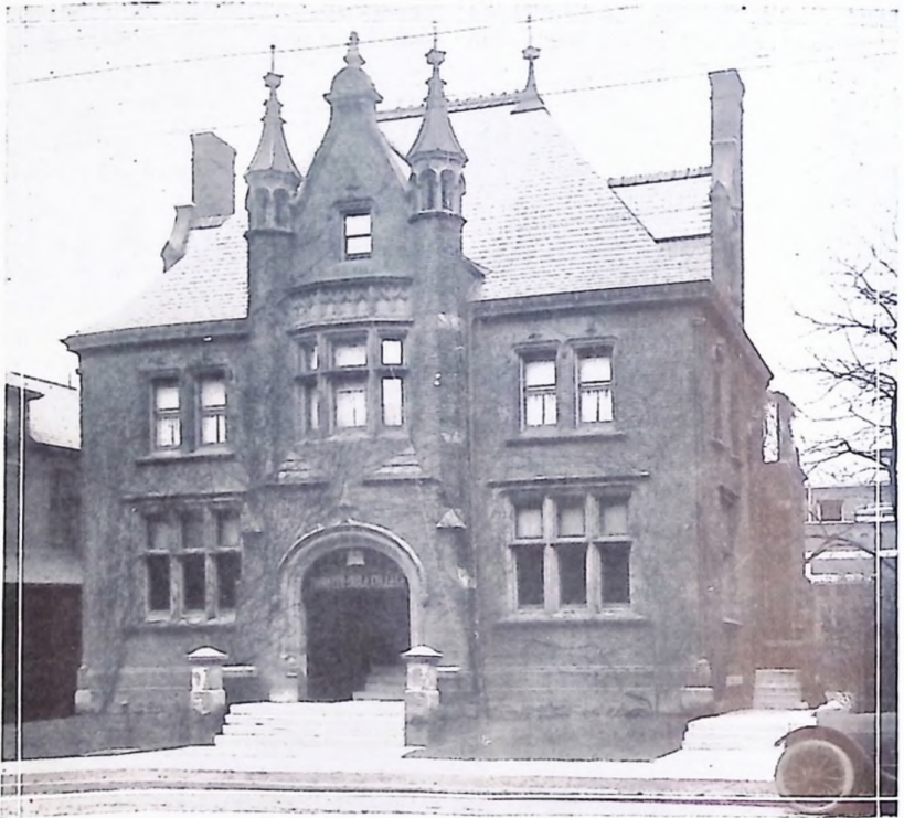
THE OLD COLLEGE BUILDING
