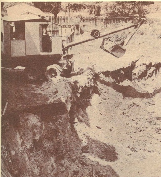
Excavating takes place a few days after the sod-turning ceremony.
